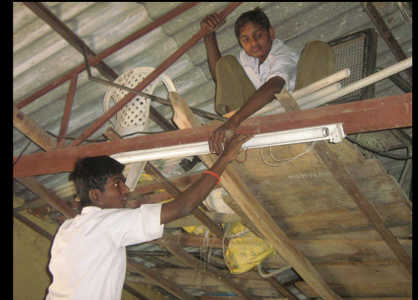
Installing classroom lights applying electrical wiring skills
