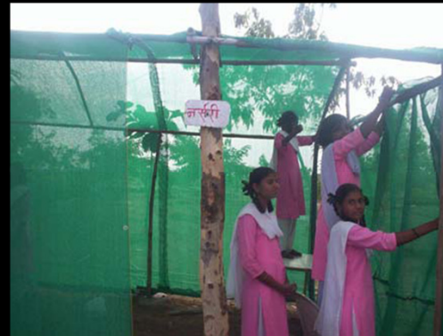
Constructing a greenhouse structure using nylon nets
