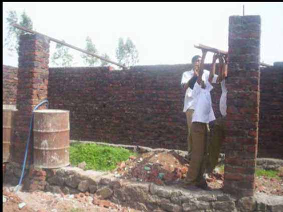
Putting together the roof for a classroom structure
